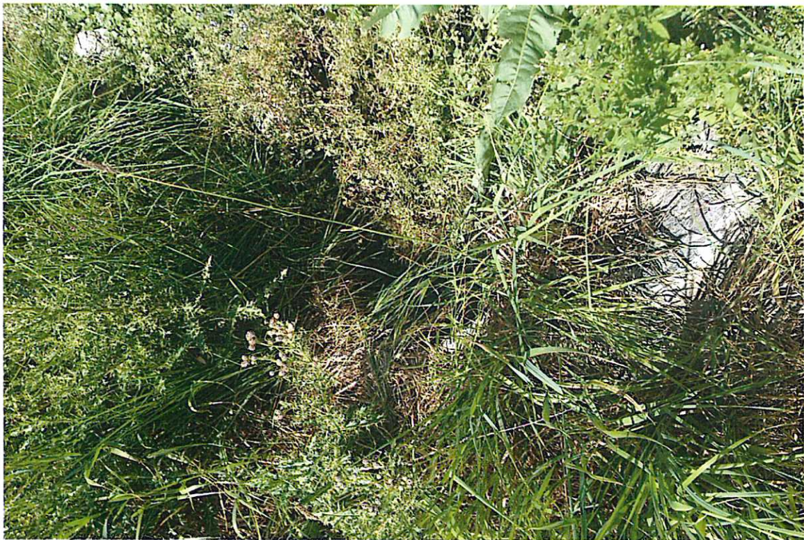
OUTFALL 8 - OUTLET INTO POND
