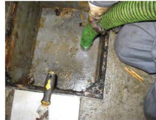
Oversee contractors for complete, correct service.
