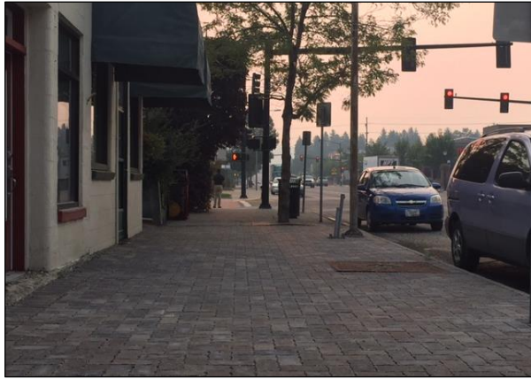
Figure 5.4-1. Permeable Interlocking Concrete Pavers in Bozeman
