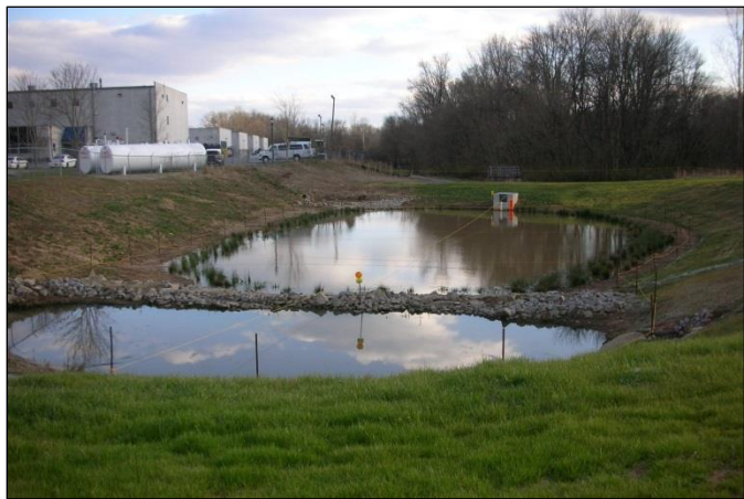
Figure 5.8-2. WDB with Permanent Pool
