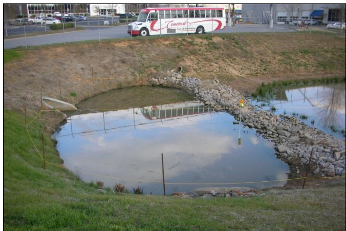
Figure 5.8-3. WDB Pretreatment Forebay
