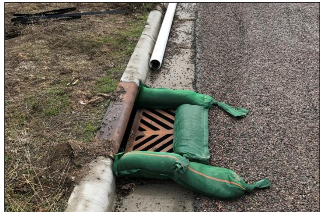
Figure 5.3-9. Inlet Protection
