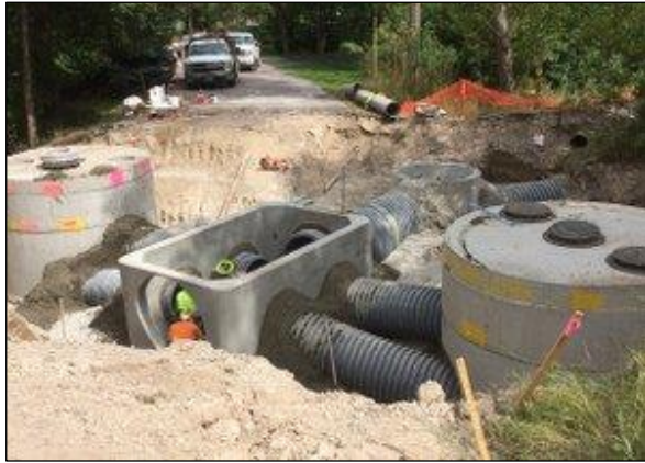
Figure 5.9-1. Proprietary Treatment Device Installation
