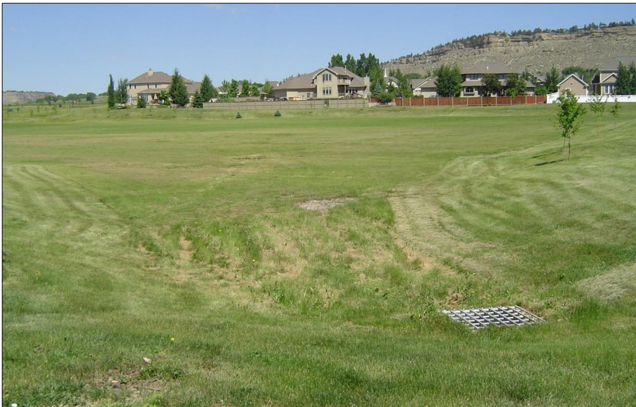
Figure 5.7-2. Detention Basin in Billings, Montana
