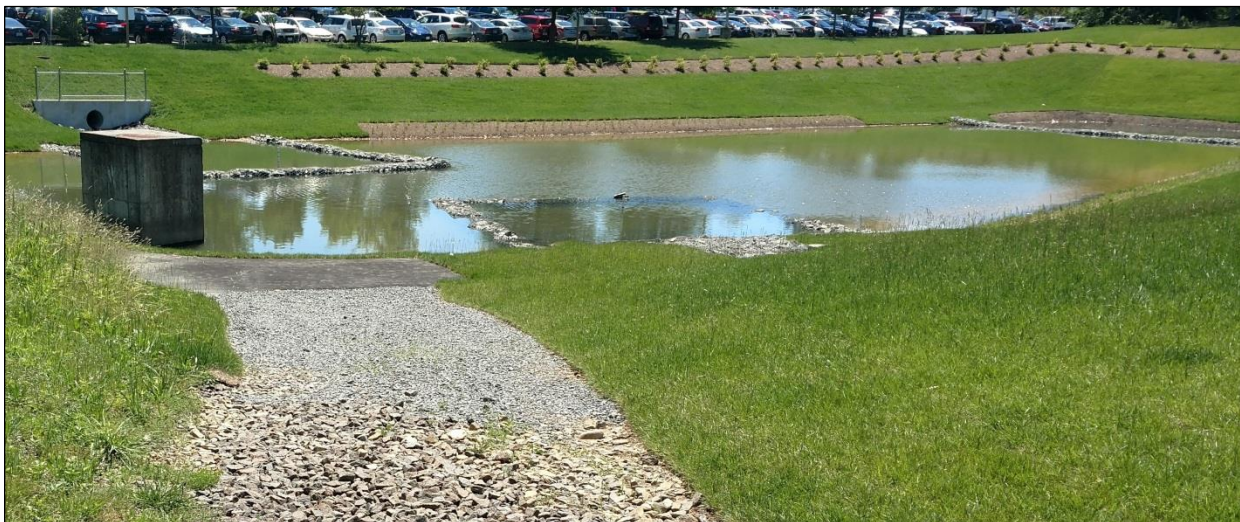
Figure 5.8-6. WDB Maintenance Access
