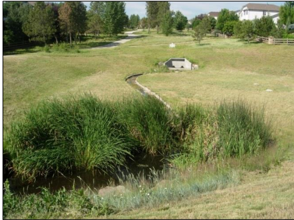
Figure 5.7-1. Extended Detention Basin Source: Courtesy of UDFCD
