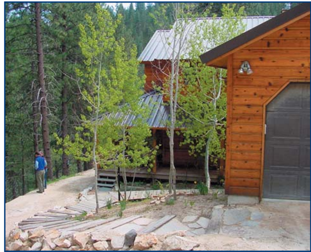
The pre-fire activities implemented by this homeowner include a maintained landscape, use of fire resistant plants, reduced vegetation around the home, and fire resistant roofing materials.
