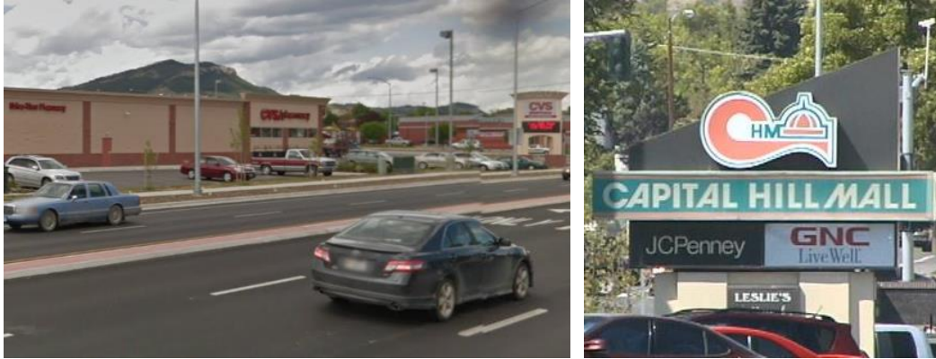
Figure 7: CVS is an anchor of Northgate Plaza Shopping Center (left). Capital Hill Mall (right) is a failing shopping area near the state capitol.
