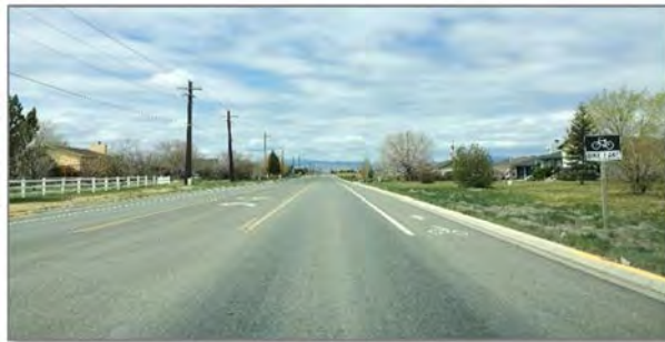
Bike lanes on Canyon Ferry Road
