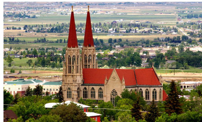
St. Helena Cathedral provides a dramatic backdrop for the Downtown. Photography by Wayne Wasilewski
